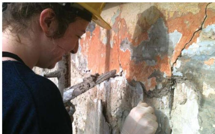
*Ceilidh Colburn 2014 ZGTF Scholar, applying mortar to the edges of damaged plaster at Qano Lani House, Gjirokastra, Albania*
