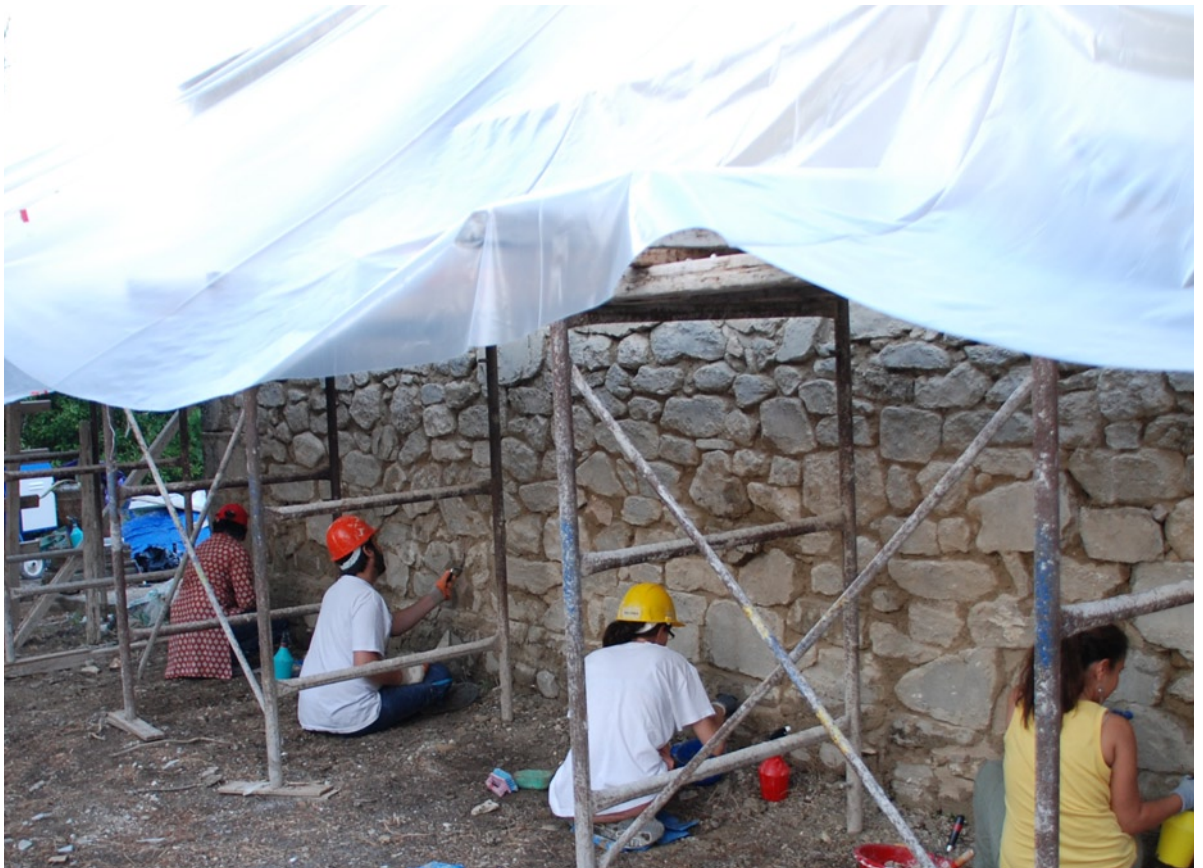
Figure 18. Repointing under the tarpaulin.
