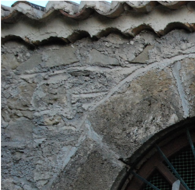
Figure 13. Evidence of cementitious mortar in use on the building.
