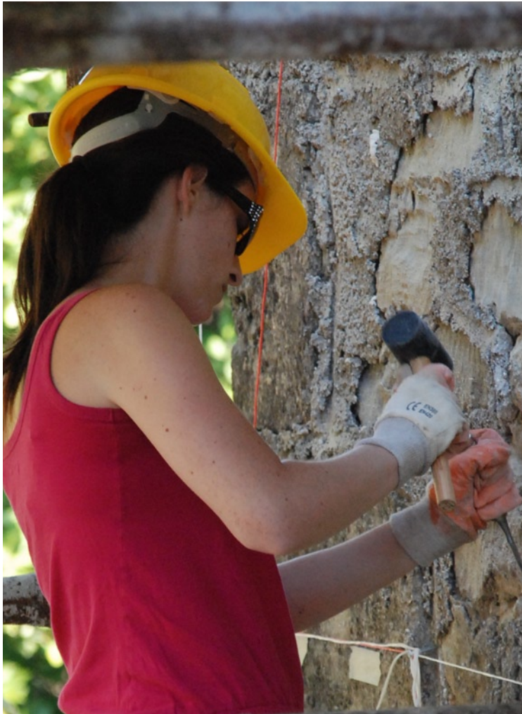
Figure 16. Removing the cement mortar.
